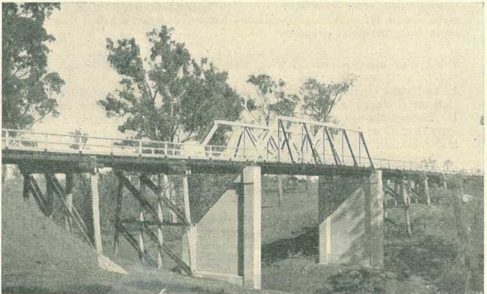
Plate 59. ALONG THE LOCKYER-DARLING DOWNS HIGHWAY.—“A” class bridge, with 8-30 feet timber spans, 1-90 feet timber and steel truss span, 20 feet between kerbs, 53 feet maximum above stream bed, constructed by the Main Roads Commission.
