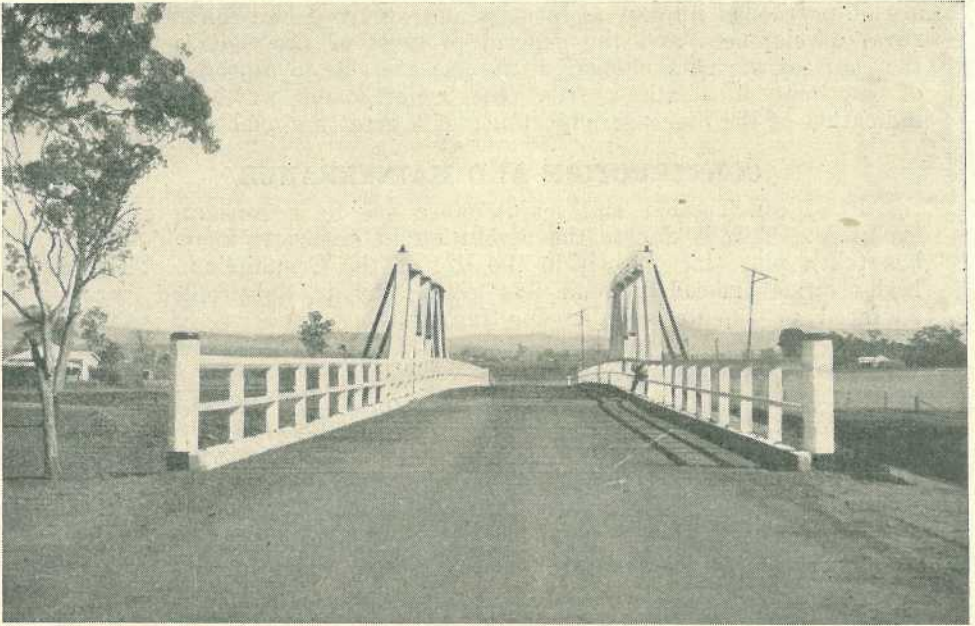
Plate 58. New Bridge over Tenthill Creek, on the Brisbane-Toowoomba Road.
