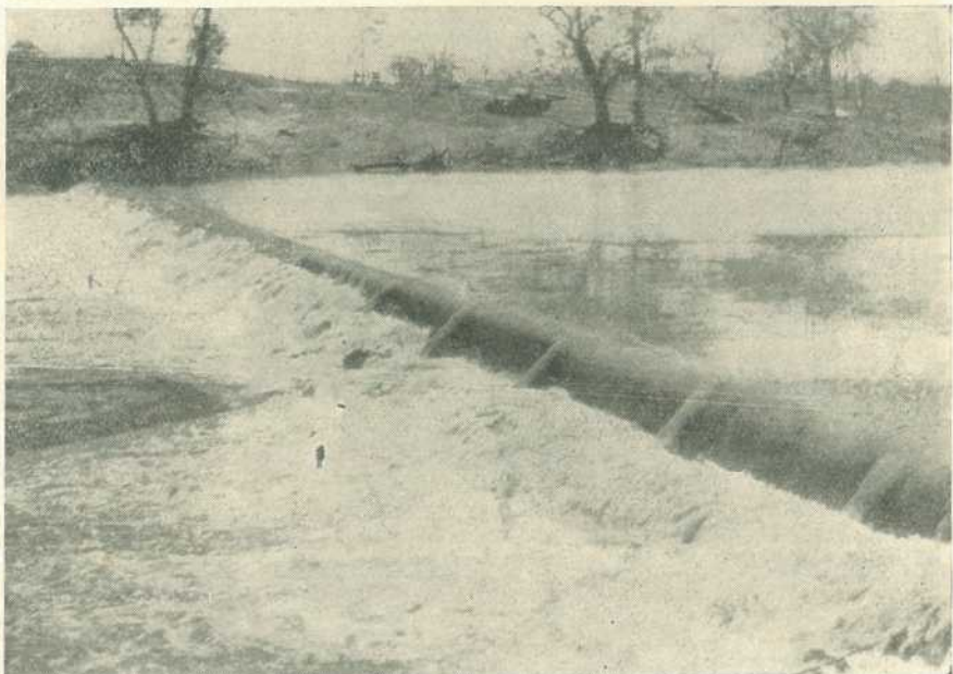
Plate 132. The weir filled to capacity.
