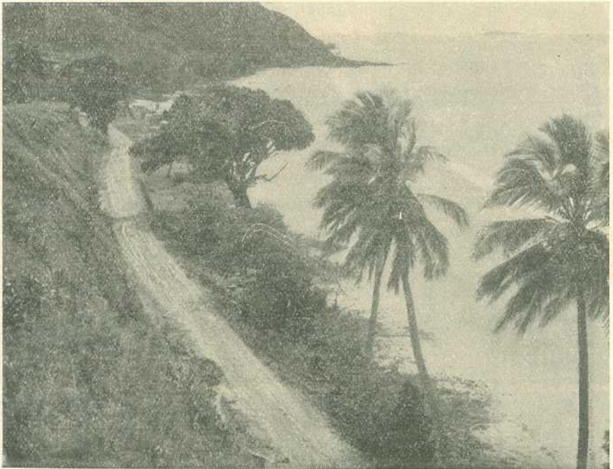
Plate 134. Access road to Bingil Bay, near Mourilyan, North Queensland.
