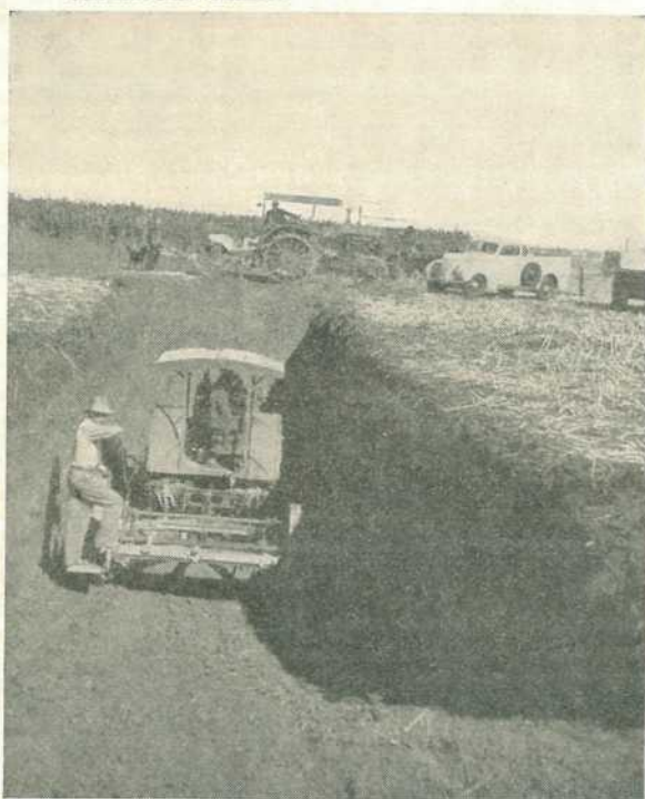
Plate 96. EXCAVATING A TRENCH SILO.
