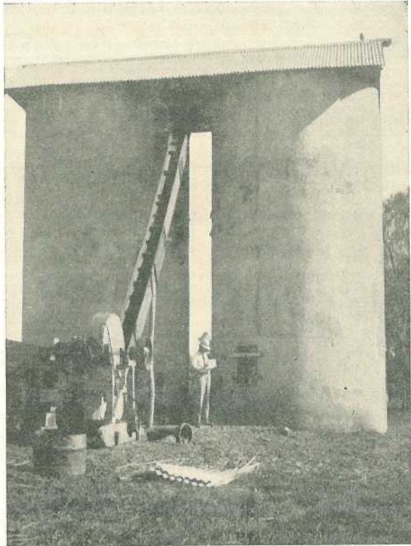
Plate 94. REINFORCED CONCRETE TWIN TOWER SILO.
