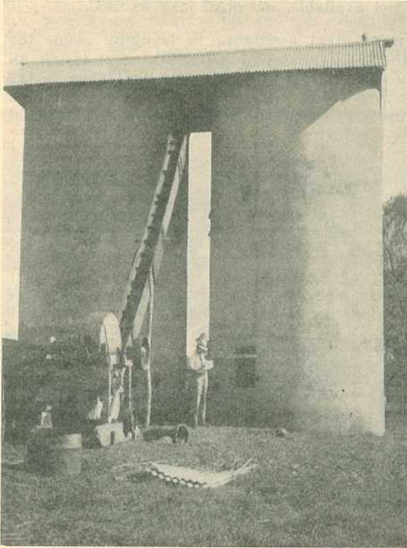
Plate 104. REINFORCED CONCRETE TWIN TOWER SILO.
