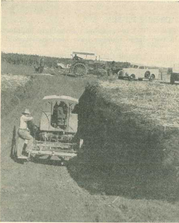
Plate 106. EXCAVATING A TRENCH SILO.
