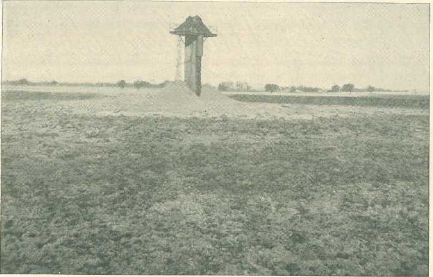
Plate 87. SUGAR BEET PULP STORAGE TANK.
