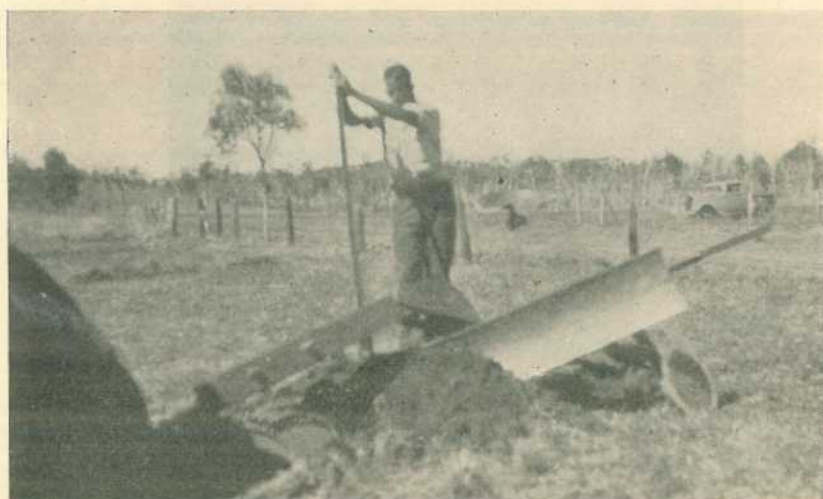
Plate 4. A Modified Grader-ditcher being Utilised for the Construction of Pasture Furrows.
