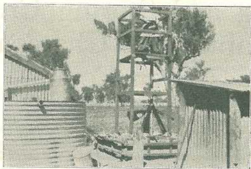
Plate 1. Building the Frame for the Combination Cooler.
