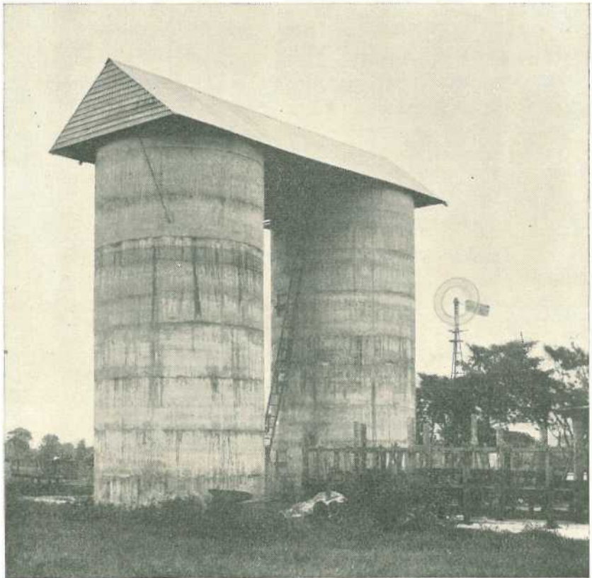
Plate 2. Completed Tower Silos.
