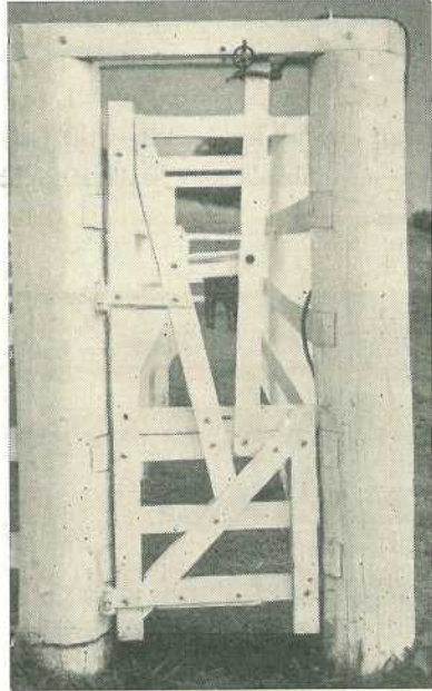
Plate 3. Gate and Bail in Closed Position.
