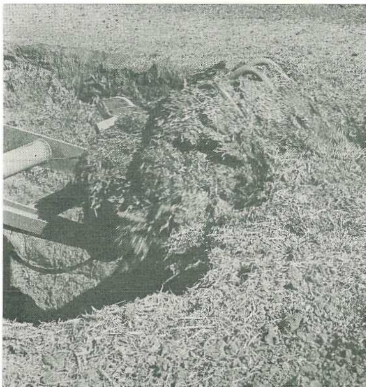
Close-up of grab at work.
