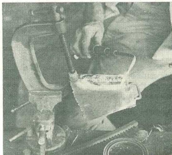
Plate 9. The bends at the top and sides of the bell are finished by hand and then the sides are held in a G-clamp while the seam is brazed.
