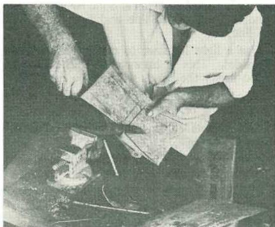
Plate 4. If the template is made from flat, galvanized iron it will last a long time. Holding one handle of the tinsnips in a vice makes cutting easier.
