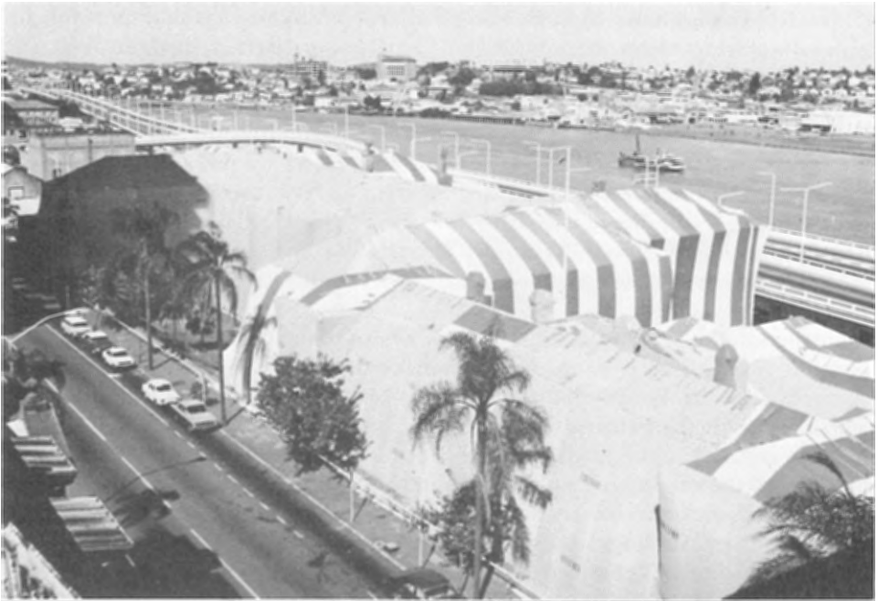
The Department's William Street offices being fumigated for West Indian termite in 1979. By this time, most branches had moved to offices in Comalco House (now State Law Building) and Mineral House, both in George Street.
