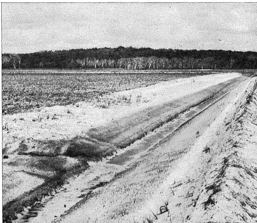
Fig. 11.—Main drain near north-eastern corner of Station.
