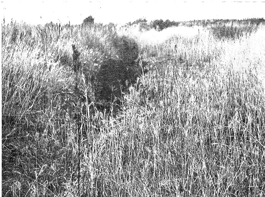
Fig. 13.—Of the 31 waterways inspected, this waterway showed the most serious gully development, including a gully 4 ft deep. Predominance of gravel in the profile suggests that the soil type was atypical and unsuited to the bare soil method. Waterway 25 in Table 2.
