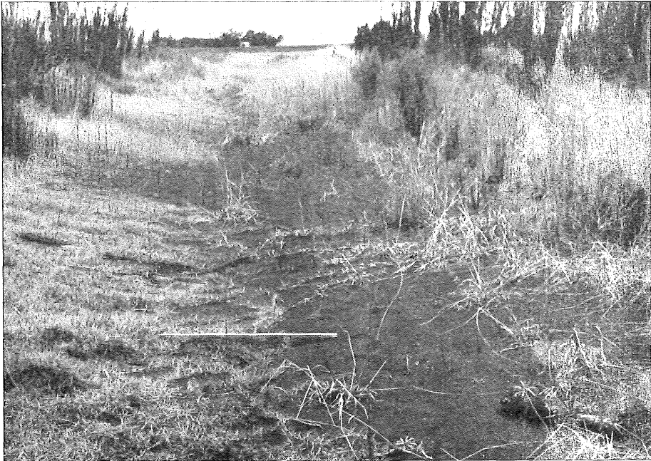
Fig. 9.—Grass was not planted in this scrub soil waterway. Some kikuyu grass plants were accidentally established on the left bank during construction and have now spread to the centre. Waterway 7 in Table 2.
