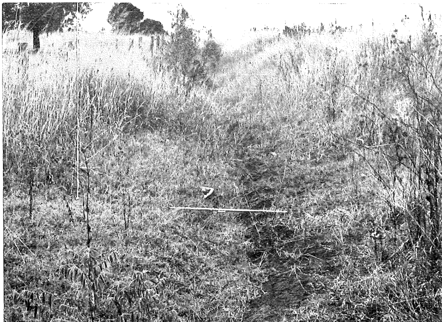
Fig. 7.—Scrub soil waterway stabilized by couch and Rhodes grasses. Centre rill 0.5–1.5 ft deep has common couch grass growing in the bottom. Photographed 2½ years after construction. Waterway 3 in Table 2.
