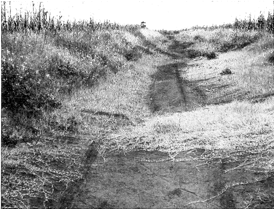
Fig. 4.—Same waterway as Fig. 1 on 30.v.1959. Waterway is still in good order and colonization has proceeded to the stage where grass will shortly meet in the centre.
