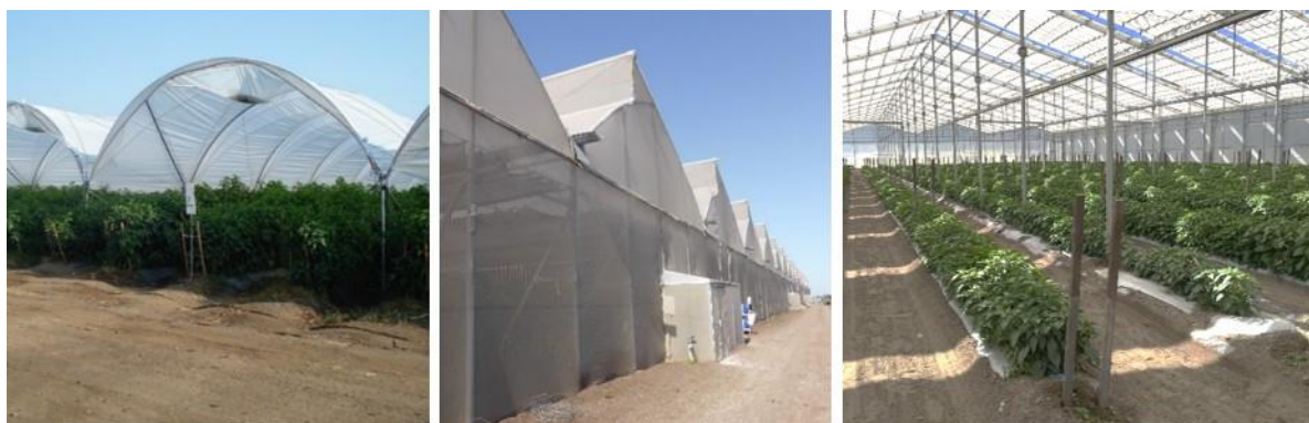
Figure 17. Images of protective structure designs included in the analysis: high poly tunnel, high passive ventilated greenhouse and retractable roof structure (Image source: Left < http://www.tierrafertil.com.mx >; centre & right: DAF).
