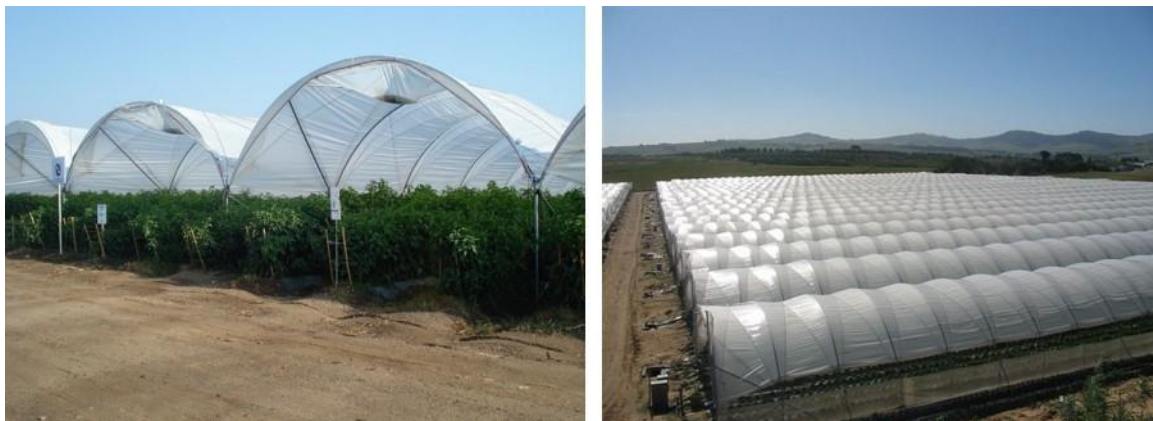
Figure 7. Examples of high tunnels as light low cost structures which are generally open or can be equipped with insect exclusion screens on the front and sides of the multispan arrangement. (Image source: < http://www.tierrafertil.com.mx > and < http://www.haygrove.com/au >).
