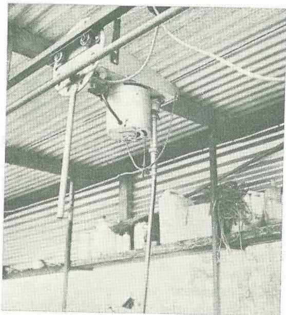
Equipment stored on a shelf under the galvanized iron roof of a race.
