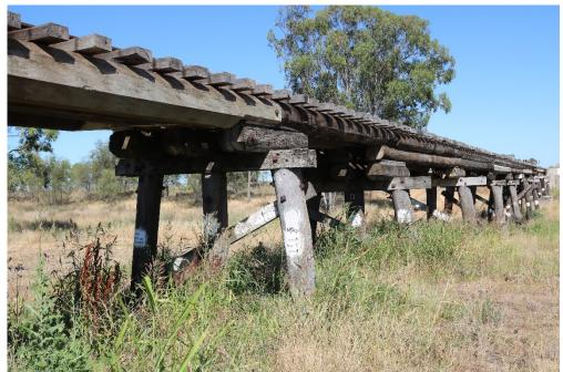
Figure 15.2. Example of a traditional timber railways bridge using timbers sections that are becoming increasingly scarce
