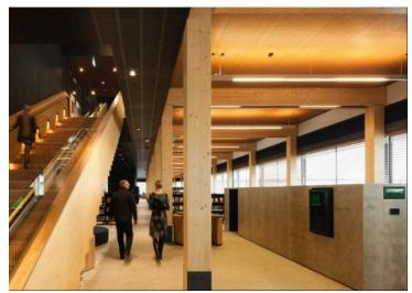
Figure 9.39. Fire designed exposed timber beams and columns at Library at the Dock, Melbourne
