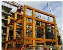
Figure 5.49. Example of Heavy HLVL timber beams and columns
