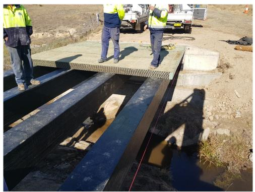
Figure 15.5. Veneer-based bridge deck and girders used for new bridge construction
