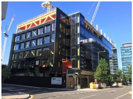
Figure 15.1. Laminated veneer lumber products featured in the recent construction of 25 King Street in Brisbane, Australia
