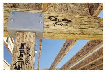
Figure 5.13. Parallam® PSL beams and columns
