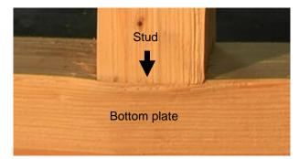
Figure 5.40. Illustration of perpendicular to grain crushing of bottom plate due to stud
