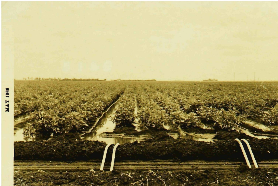
Plate 3. Cotton being grown under irrigation in the Brookstead District.
