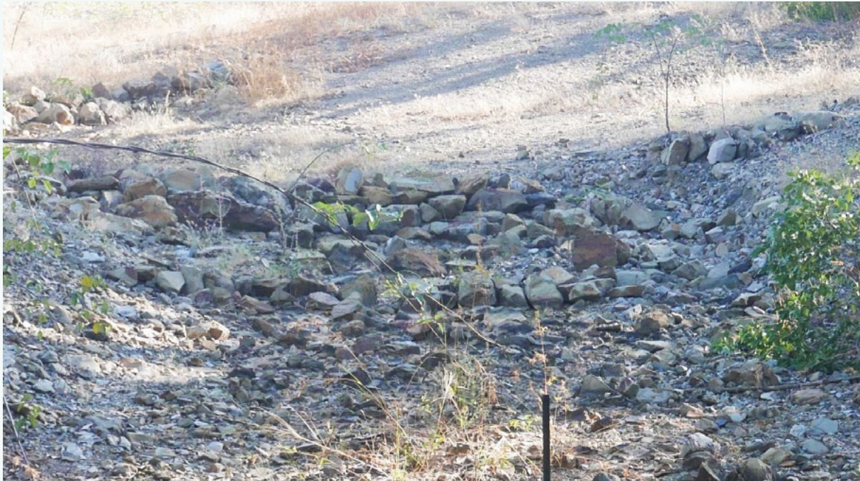
Figure 26: This gully in the Normanby River catchment was reshaped and capped with rock in 2016.
