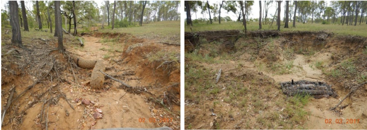
Figure 16. An illustration of known failure mechanisms for porous check dams. In these cases, the failures were attributed to the catchment areas being too large given the high rainfall and shallow soil. In addition, the coir log check dam was not adequately secured, and the material has poor durability (left). The ends of the timber and wire check dam were either not keyed into the bank or wrapped up the bank to above the flow level (right).
