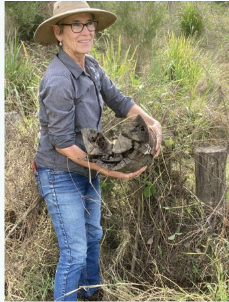
Figure 32. A pile in 2021 that was installed 6 years previously and is now rotten
