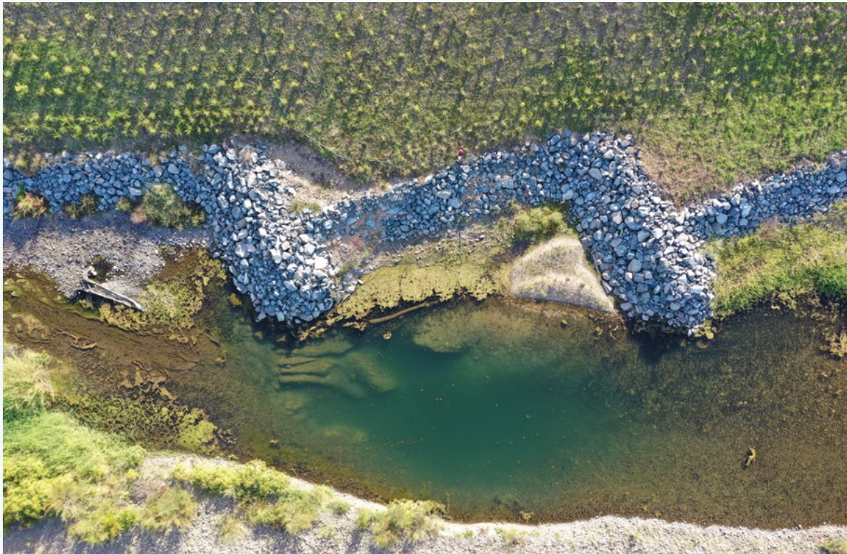
Figure 34: Rock groynes and bank reshaping at a site on the O’Connell River in July 2021, 9 months after construction (direction of flow from left to right). The scour pool shown developed over the 2020–21 wet season and had a maximum depth of 2.5 m. Note also the deposition of gravels on the upstream side of the right-hand groyne. Design equations required a median rock diameter for the groynes of 1.1 m. The groynes were keyed into the bed by 2.5 m based on the predicted bed scour depth at the design flowrate (which had a 1:20 year recurrence interval). The crest height of the groynes was approximately 0.6 m above the opposite bar surface so that the reshaped bank was relatively more protected from scour. Rock revetment was installed between the groynes to reduce the risk of groynes being outflanked. The reshaped bank was fenced and revegetated in November–December 2020.
