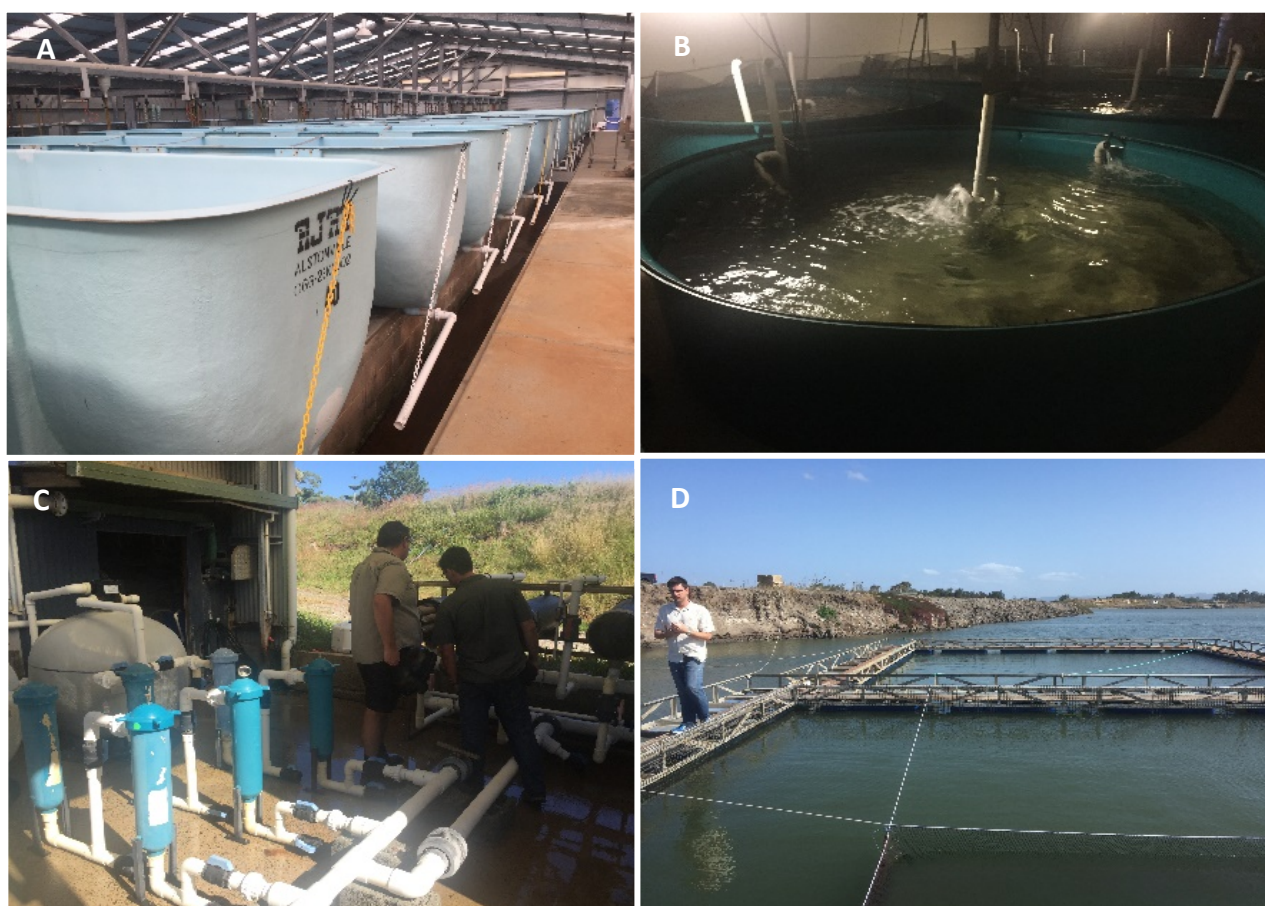
Figure 1. Facilities at RPPF used during the project. A. Parabolic tanks (10,000 L, 20,000 L). B. Round tanks (6,000 L). C. Hatchery water filtration system. D. Cages in landlocked saline lake.
