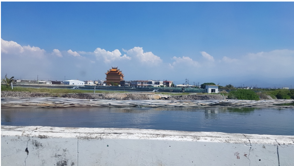
Figure 10: Concrete walled ponds in Ping Tung County
