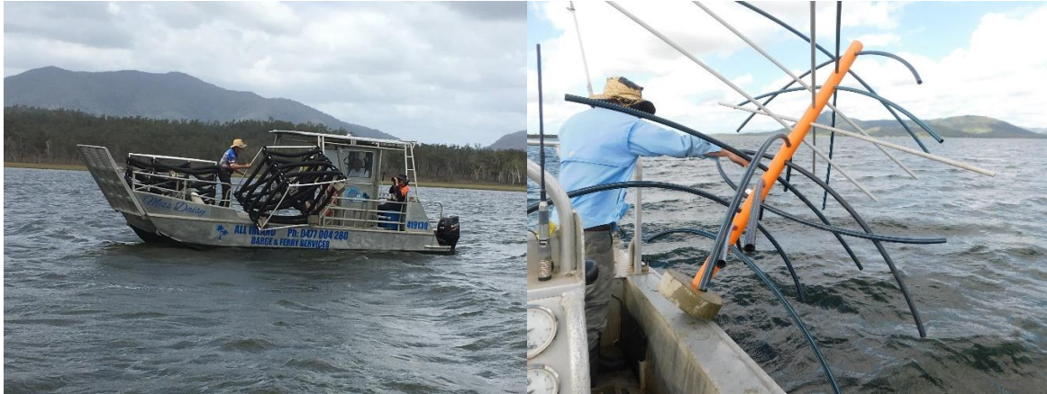
Figure 5 Ballasted Georgia Cube being deployed from side of barge (at left), and synthetic tree being deployed from the gunwale of the smaller DAF vessel (at right).
