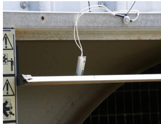
Figure 21: Mercury tilt switch with fan turned on (shutters open, switch open)
