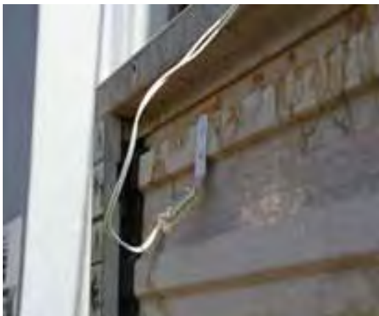
Figure 18: Mercury tilt switch with fan turned off (shutters closed, switch closed)
