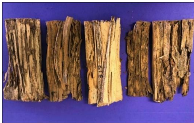
Fig. 6. The majority of the softwood feeder blocks were substantially damaged
