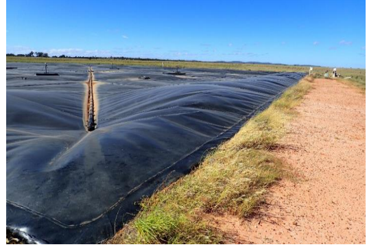
Figure 6. RCM-designed, heated, stirred, in-ground hybrid CAP.
