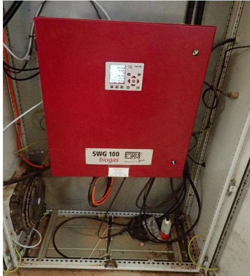
Figure 1. Upgraded biogas analysis system (MRU SWG 100 biogas) supplied by Phoenix Instrumentation.
