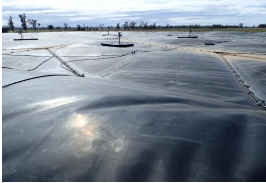
Figure 5. Hybrid CAP cover showing the stirrer and air injection locations.
