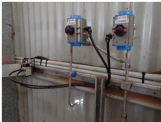
Figure 3. Pneumatically operated valves with remote solenoids to control biogas flow from the two sampling points to the analyser.
