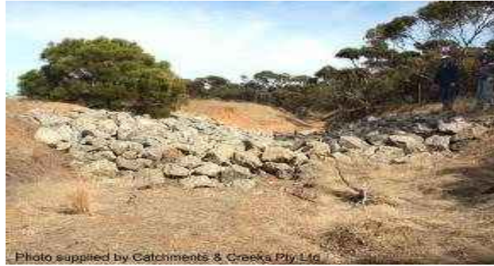
Figure 21. Rock weir and drop structure used to stabilise gullies.
