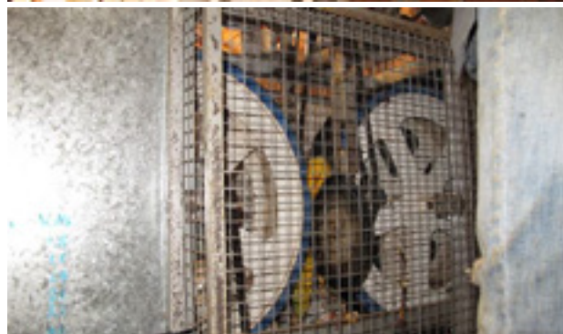
Figure 15. Pod alignment conveyor which feed pods into the pod splitter
