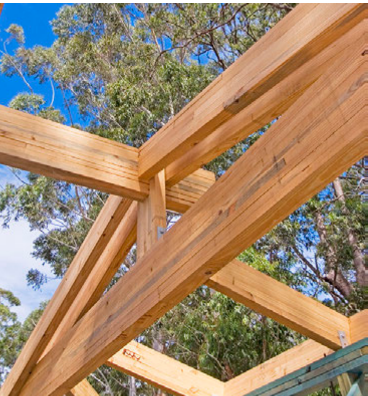
Glulam beams used in house construction (photograph courtesy of Hyne Timber)
