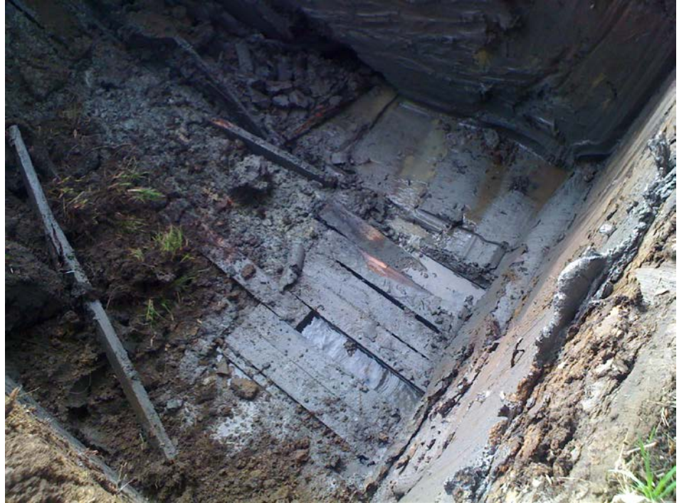
Wooden sewer tunnel
