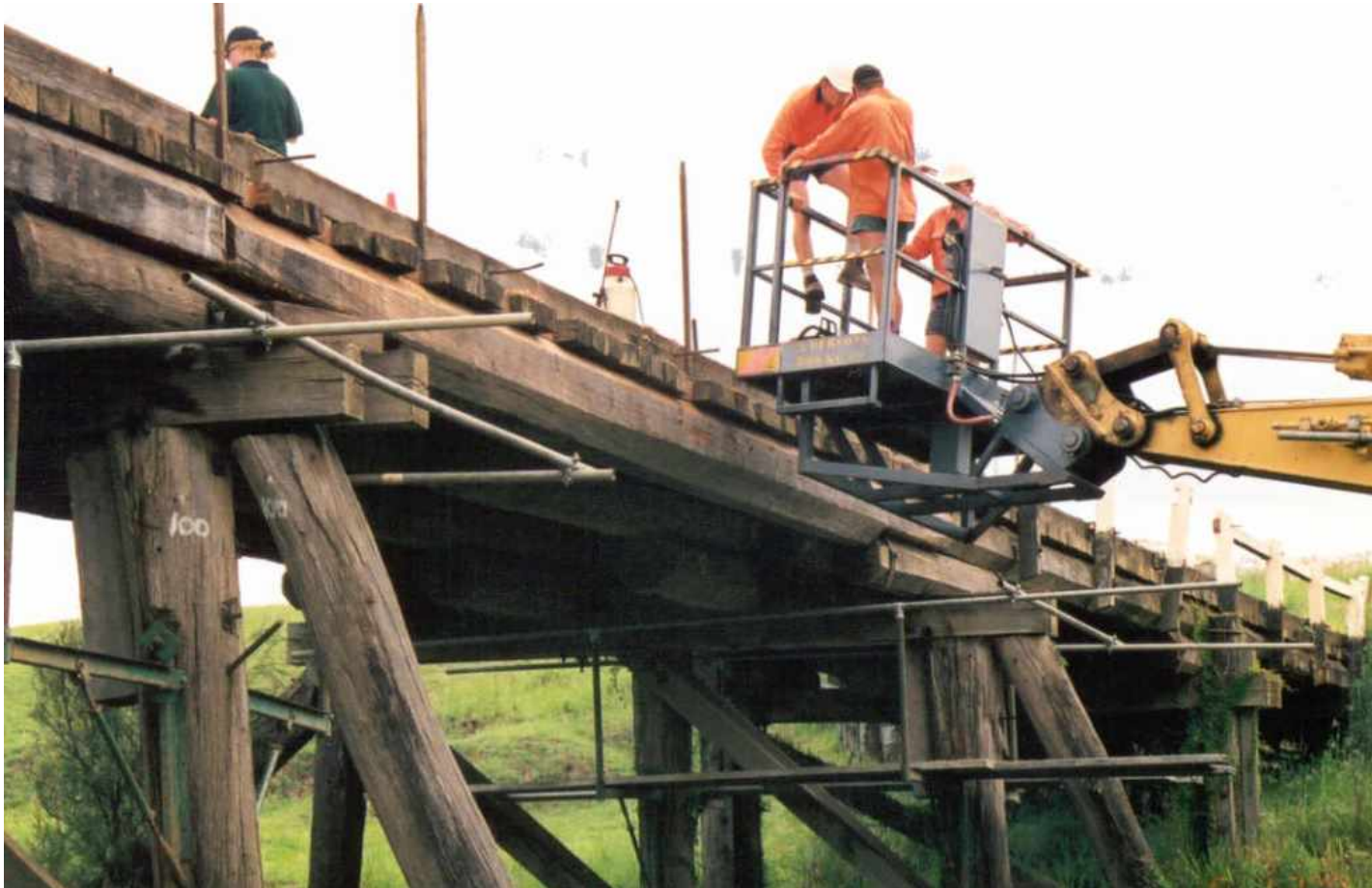
Heritage listed timber bridge, client: Beaudesert Regional Council
