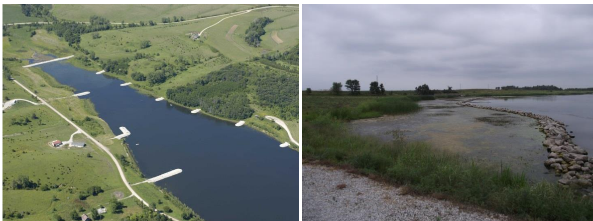
A series of rock groins have been installed to reduced wind erosion, provide additional habitat for fish and improve angler access (images NGP)
