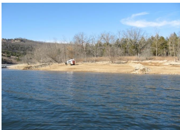
Rock and gravel fences installed to increase habitat complexity and enable access to finer gravel substrate for spawning nests (images MDC)
