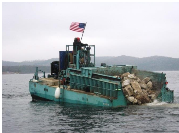
Rock mounds built in a Nebraskan reservoir and constructing a rocky reef in Table Rock Lake, Missouri (images NPG and MDC respectively)
