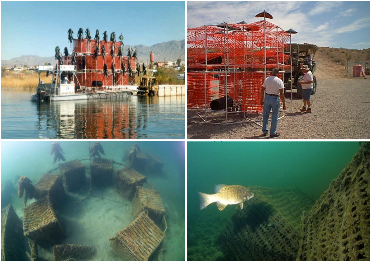
A range of fish habitat structures created from snow fencing wrapped around a PVC frame. Note the thick algal growth in the lower two images (Images BLM and A. Norris)
