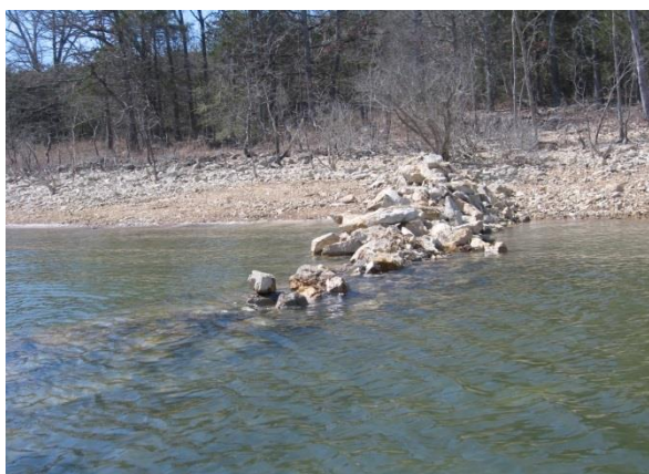
Rock and gravel fences installed to increase habitat complexity and enable access to finer gravel substrate for spawning nests (images MDC)
