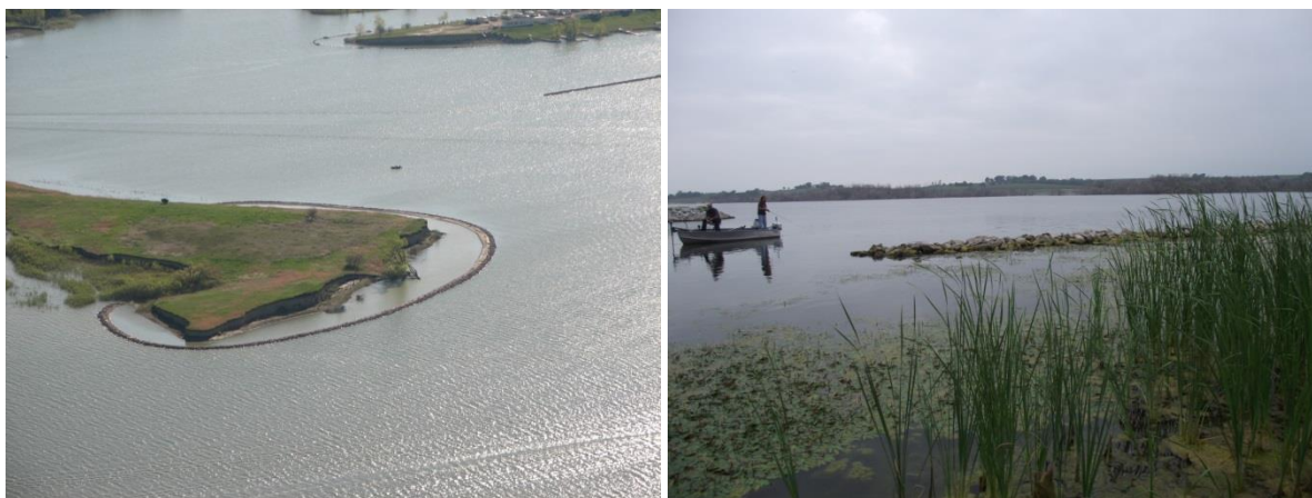
Off-shore breakwaters protect the shoreline from erosion and create additional fish habitat and protected areas for aquatic vegetation to establish (images NGP and A. Norris)
