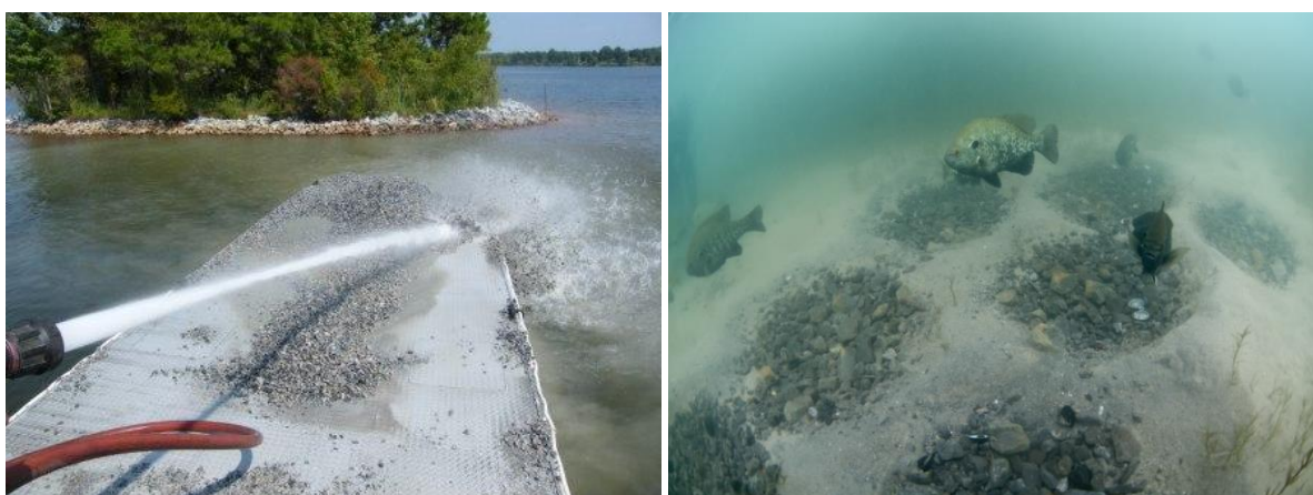
Deploying gravel off a barge with a high power hose and redear sunfish nests in a gravel bed (images NCWRC)
