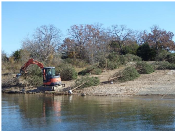
Staging weighted trees ready for loading onto the habitat barge.
