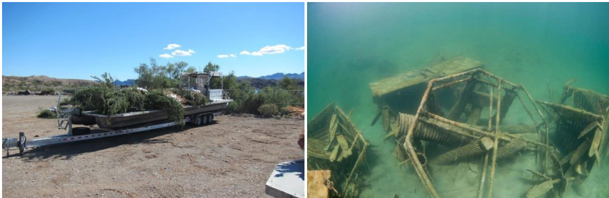
Brush piles loaded on the barge ready to be deployed by volunteer. PVC and snow-fence structure starting to break down. Boat anchors can have a large impact on these structures.
