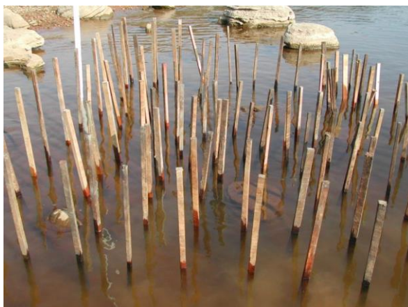
Pre-fabricated stake beds to provide vertical structure for fish (images PFBC)
