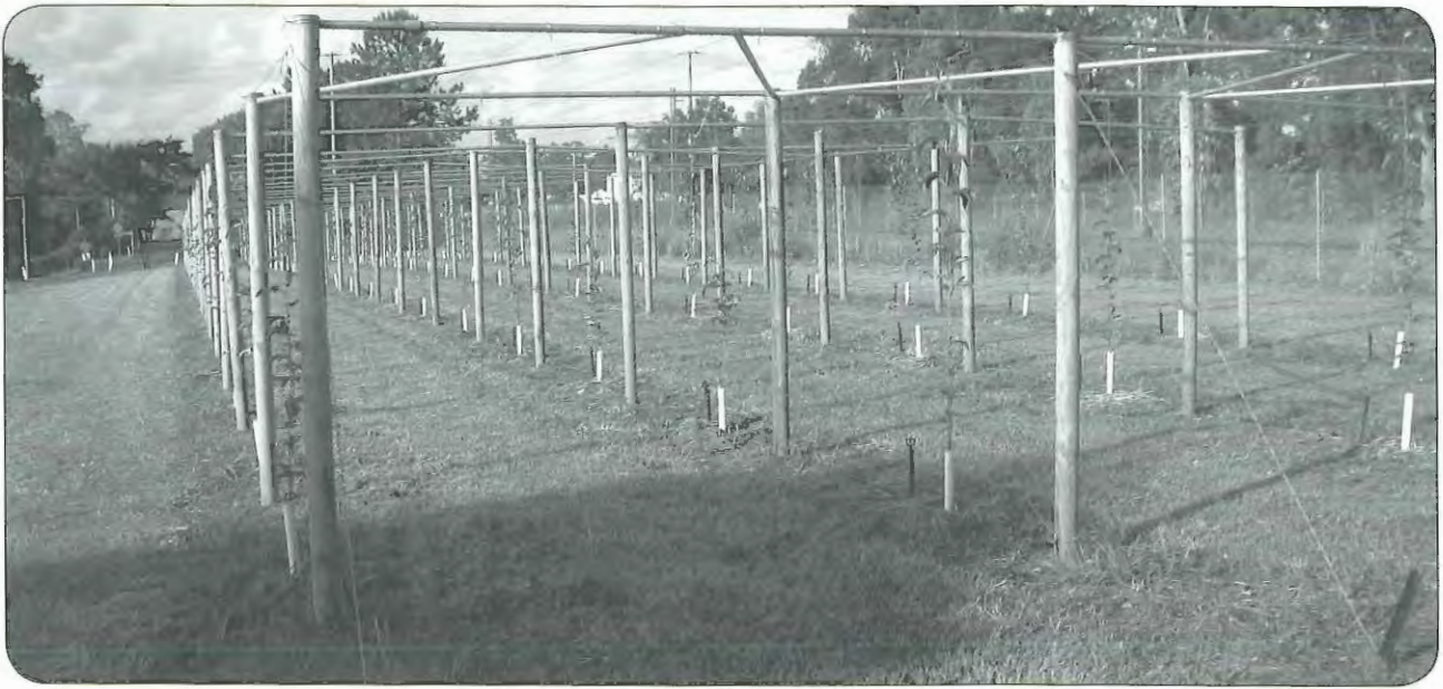
Figure 6.5 Metal pipes and guy wires to star picket anchors have been used to strengthen this pergola structure
