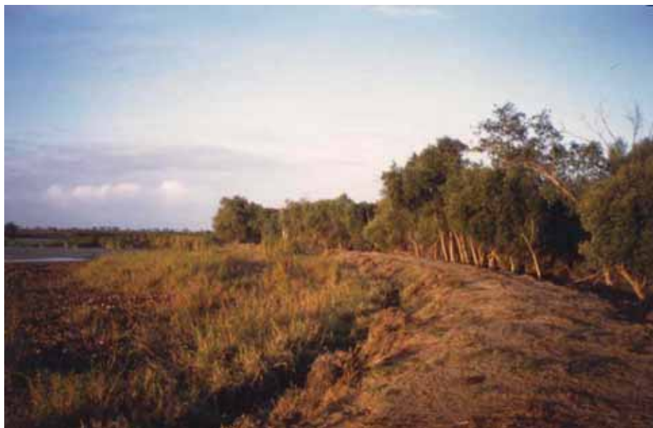
Figure 4.2 A bund wall against an Avicennia community on Plantation Creek
