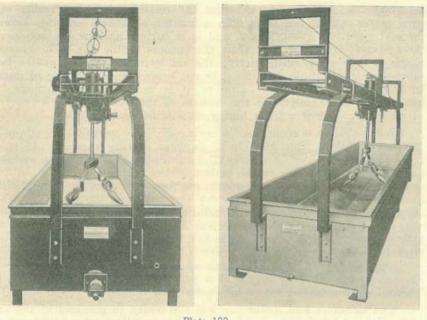
Plate 133. Two Views of Travelling Agitator and Curd Stirrer.
