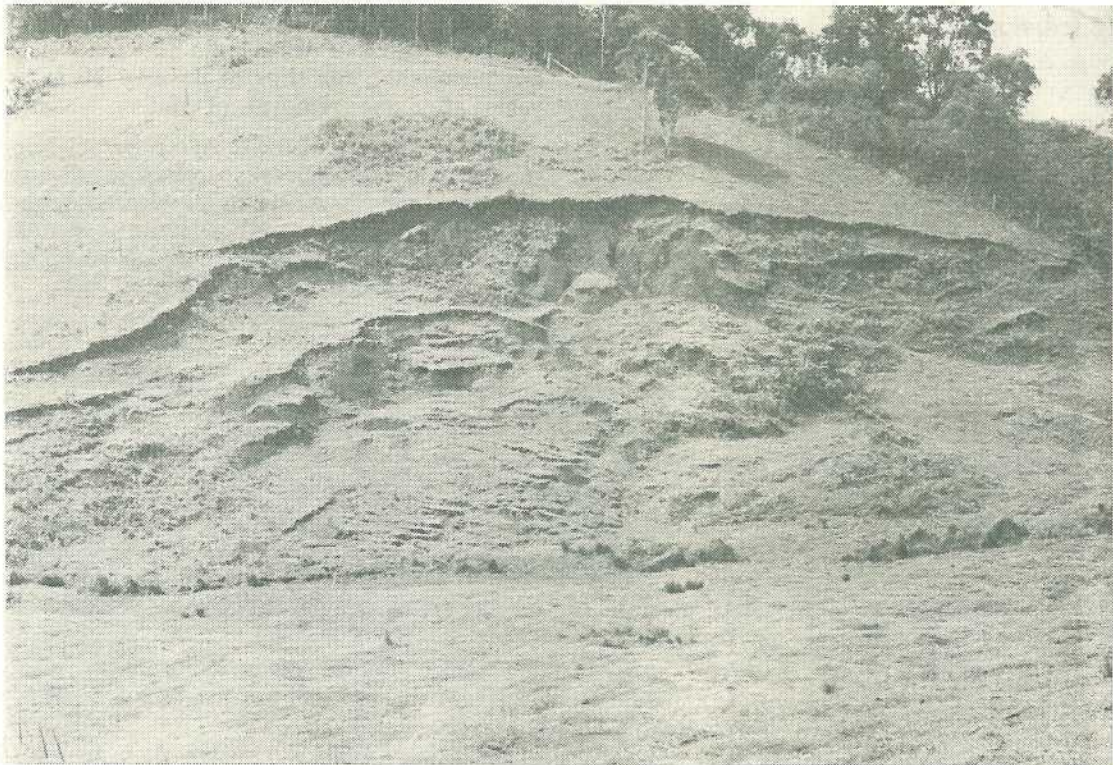
A slump in the Montville area.
