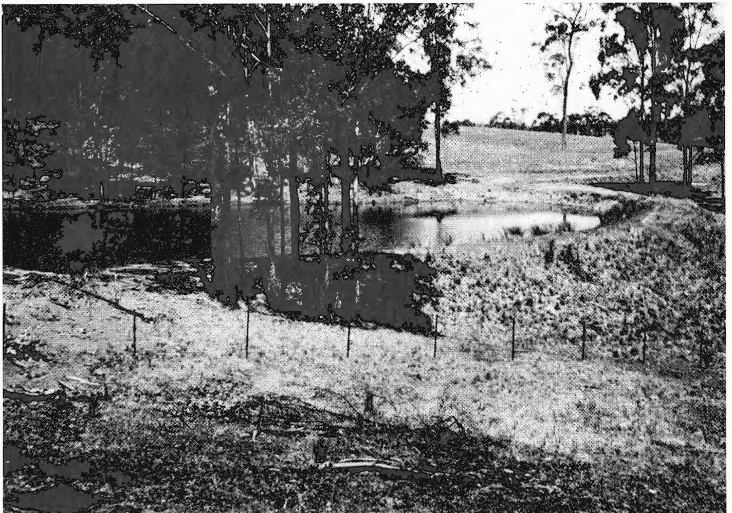
Plate 3. Trees should not be planted on dam walls as they may affect the dam seal and attract stock onto the bank.
